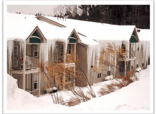
**Figure 1: Fiberglass insulated structure along with a combination of several other icicle causing factors.**
