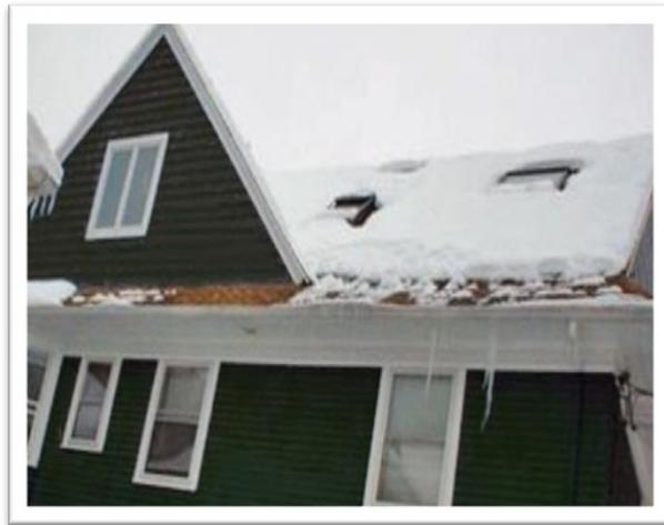
Figure 6: Reverse ice damming can be identified by lack of snow on the overhangs, but not the remainder of the roof.
